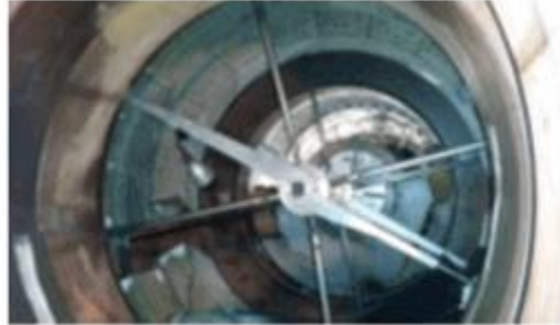
Alignment of casings
