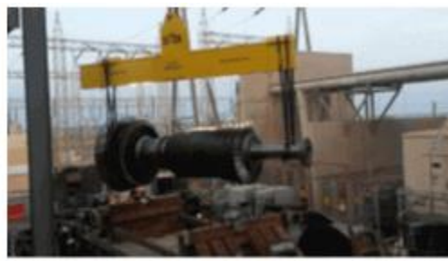
Rigging of new rotor
