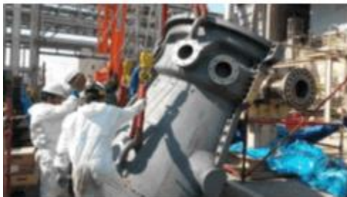
Installation of Mid Compressor Casing
