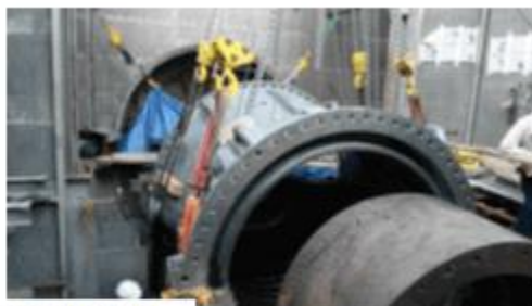
Installation of Mid Compressor Casing
