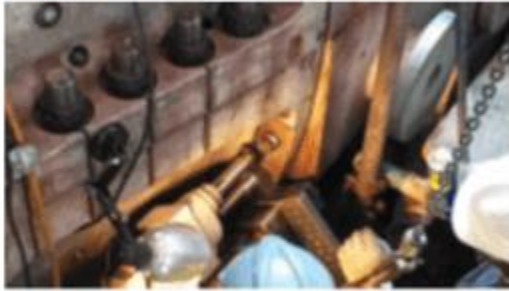
Re-doweling in progress
